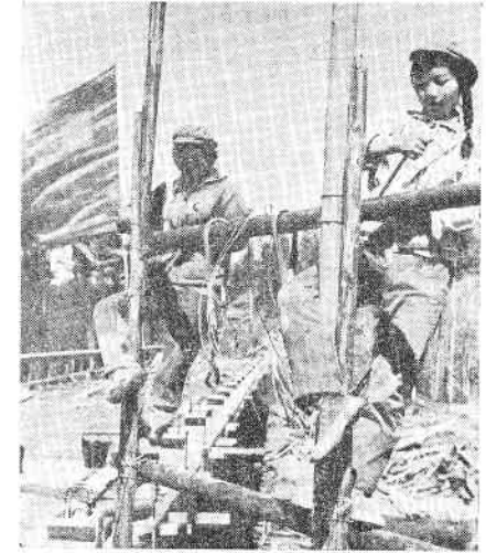
At the bridge construction site.
