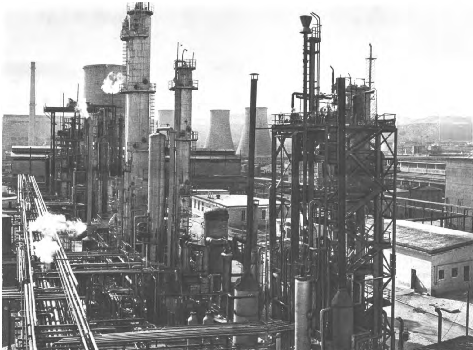
Up-to-date equipment for the chemical industry.
