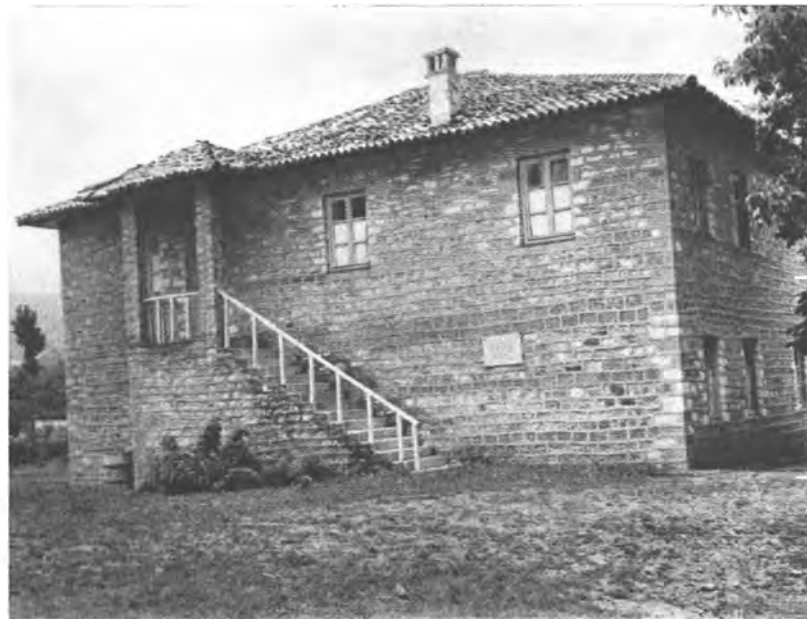
It was in this house at the village of Peza in the Tirana District that the First National Liberation Conference was held on September 16,
