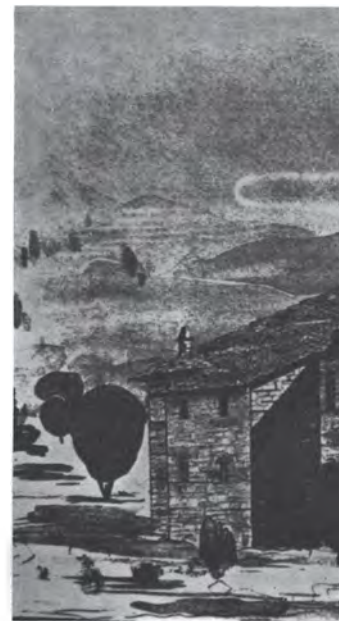
At the village of Frashëri where brothers Abdyl, Sami and Naim Frashëri, distinguished men of our National Revival, were born, their house is being reconstructed to stand out as a museum. It is being rebuilt on the site where the old house stood and the excavations have unearthed the foundation, staircase and portal of the old house built some two hundred years ago.
