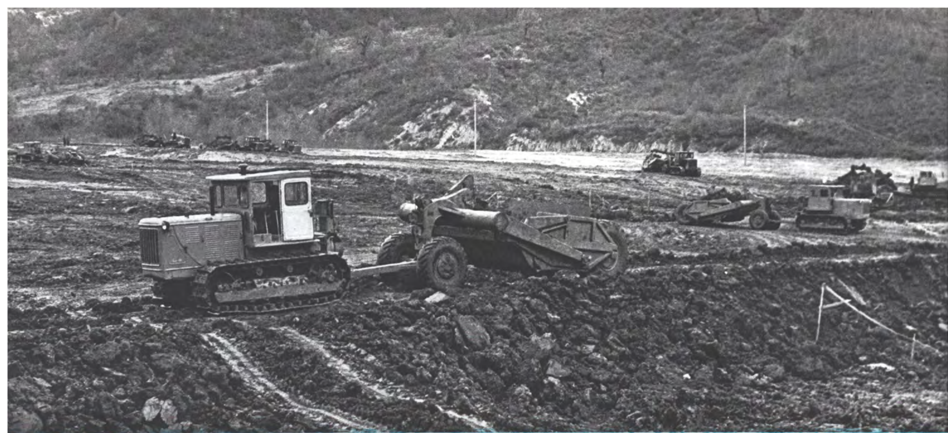
The Deep Oil Processing Plant is being built here in Ballsh.
