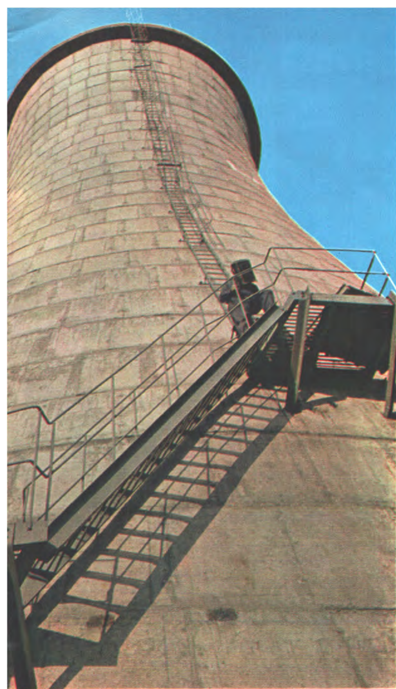
The thermoelectric station (TEC) of Korça.
