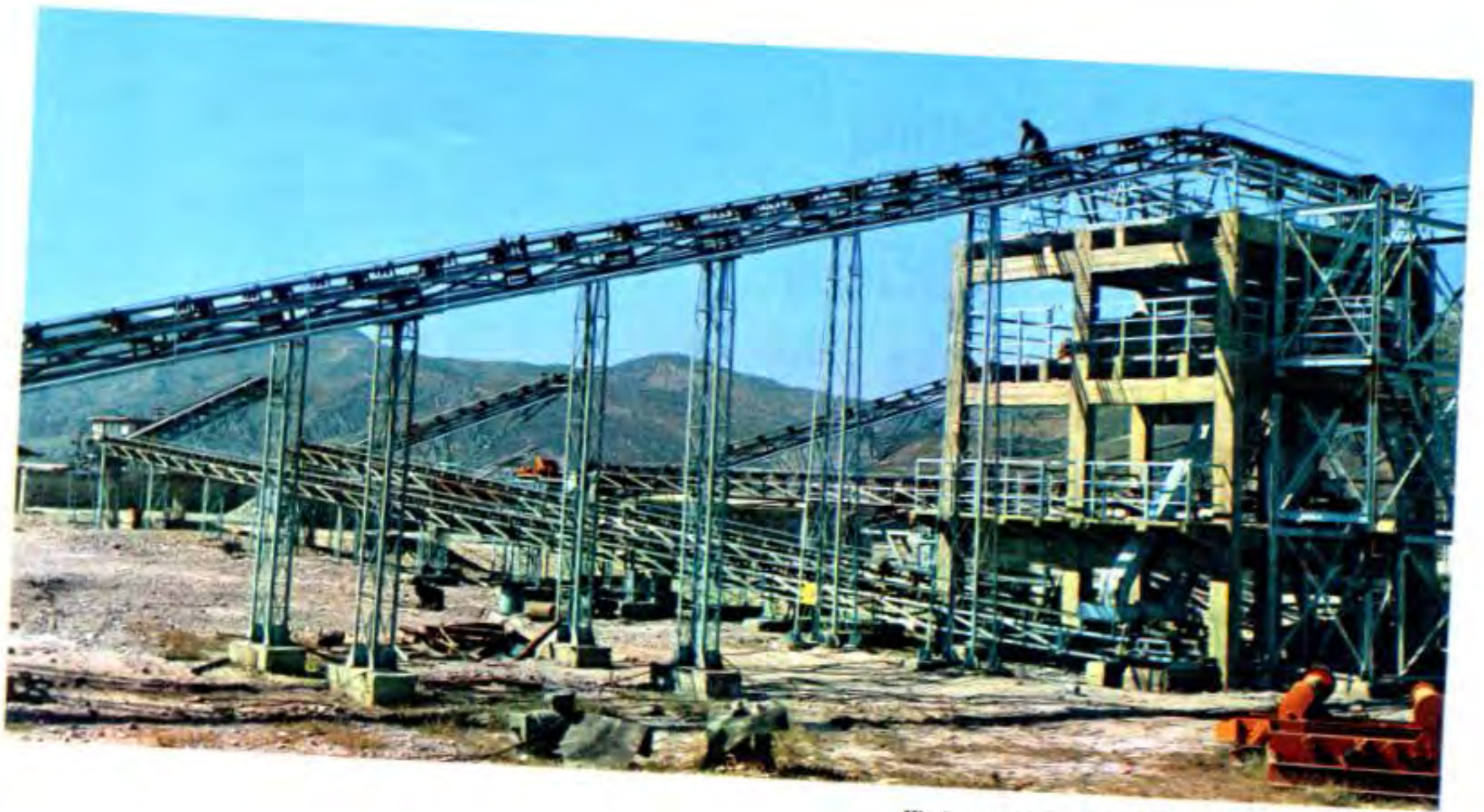
Work has begun on setting up the complex of buildings.
