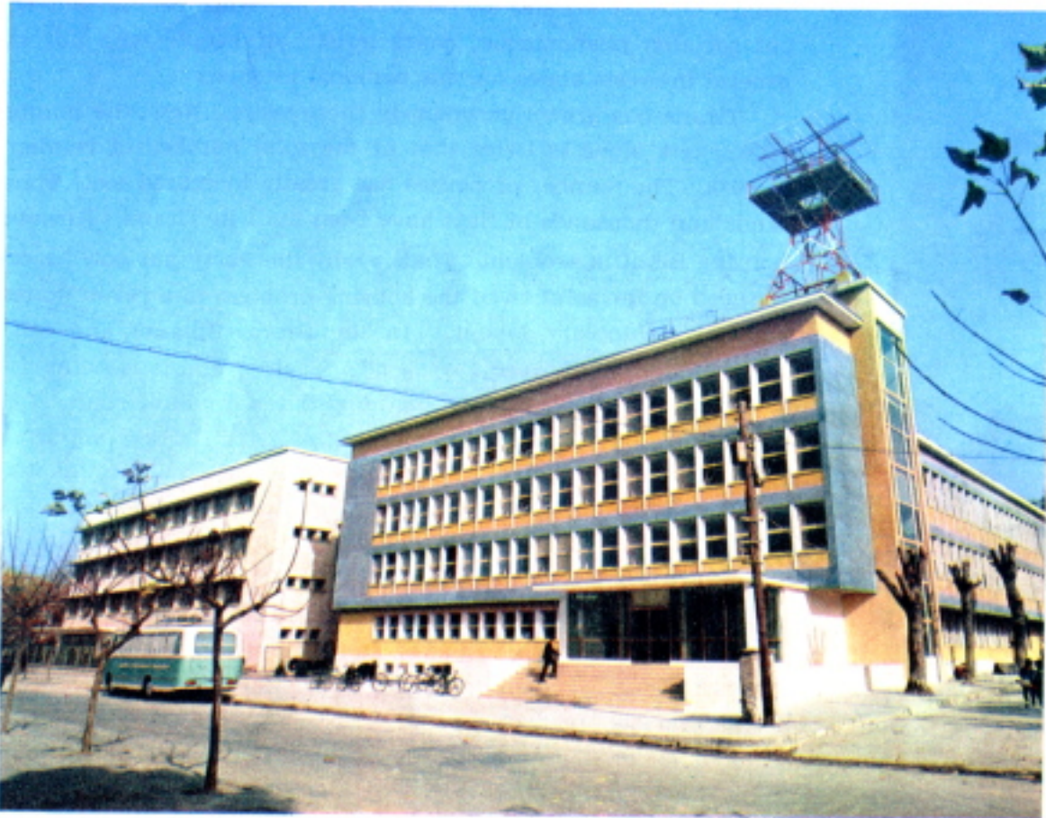
The Albanian television building constructed in recent months.
