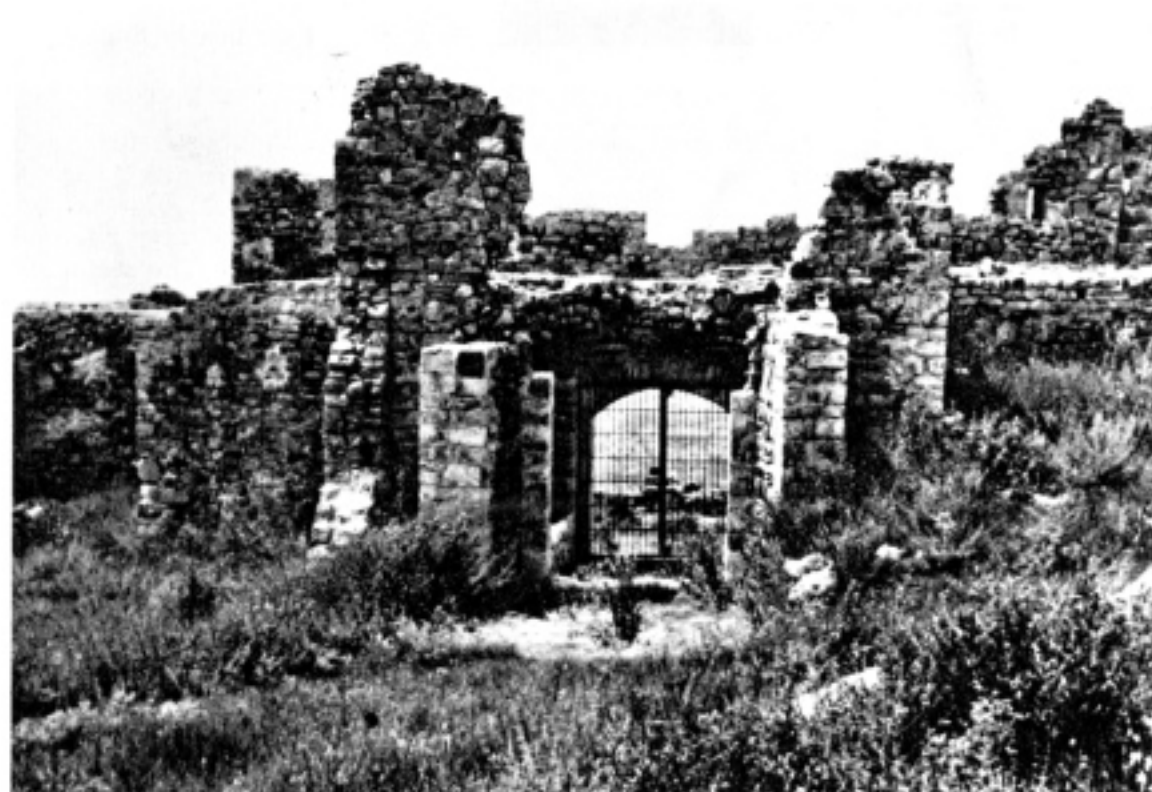
Interior view of one of the three gates of the castle built in the 11-th century bearing traces of Venetian and Turkish restoration.
