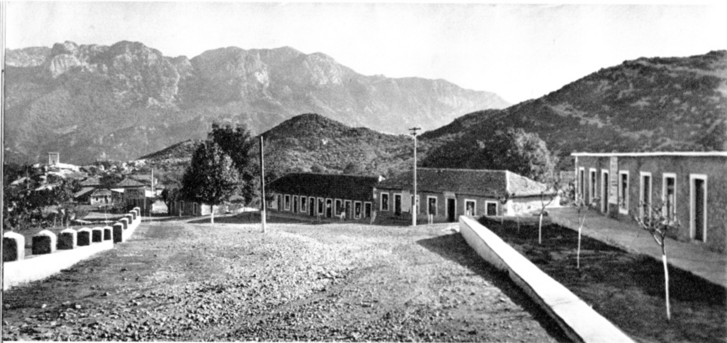
New buildings in the Vrith Agricultural Cooperative, Shkodra District.
